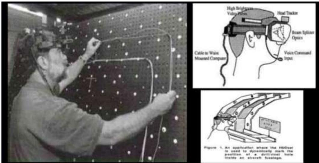
Figure 6 - First smart glasses application in Boeing by T. P. Caudell and D. W. Mizell (adapted from : <https://www.timetoast.com/timelines/educacion-oblicua> retrieved on November 26, 2020)
